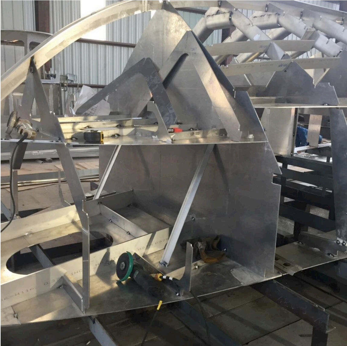
Installation of Forward Frames
