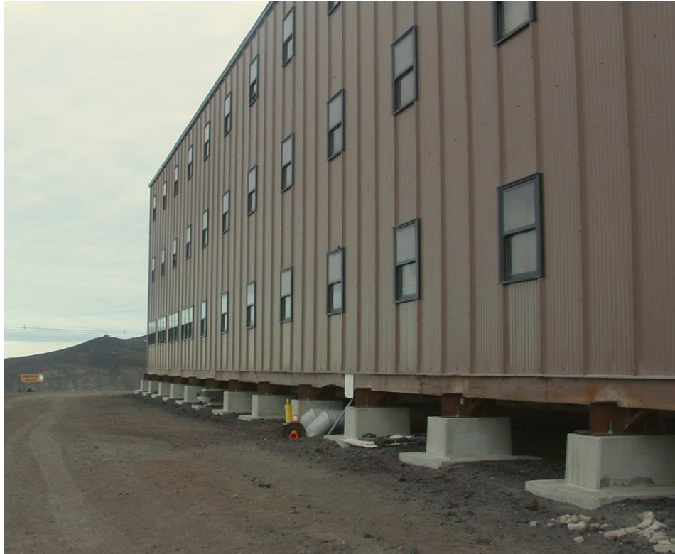
Photo 3 – Existing Precast Spread Footings Supporting Structure
