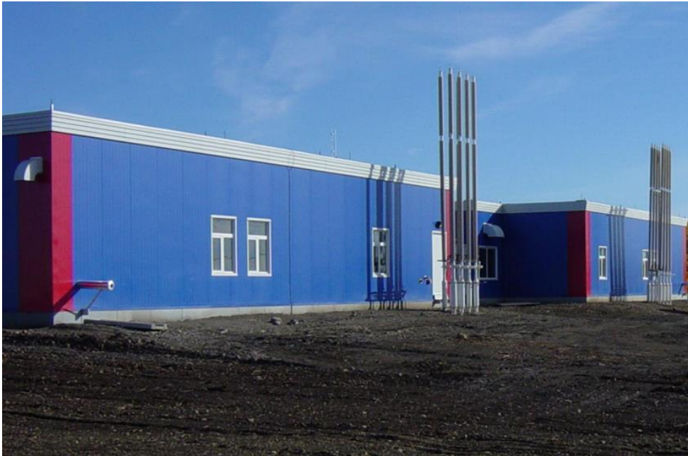
Photo 1 –Slab on Grade Supported Structure with Thermal Syphons
