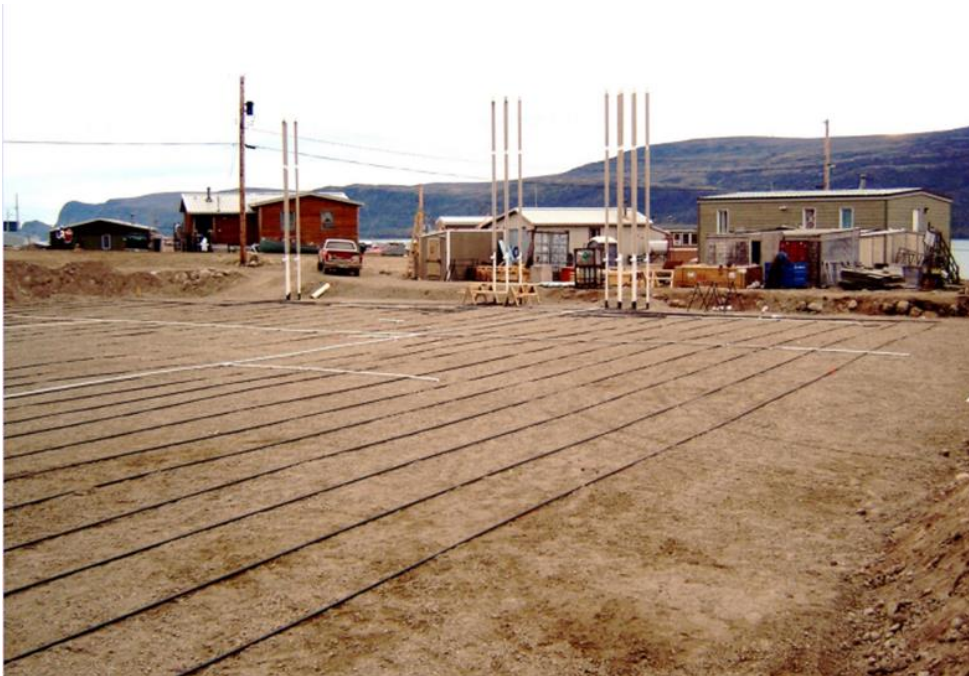
Photo 2 – Installation of Thermal Syphon System
